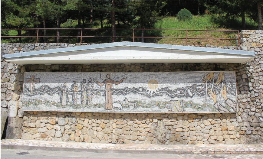
Figure 14. The Convent and the Parish Church of Saint John the Baptist, Kraljeva Sutjeska: scenes from the life of Saint Francis done by Vladimir Blažanović in 1988, mosaic on the retaining wall in the inner courtyard (2013)
